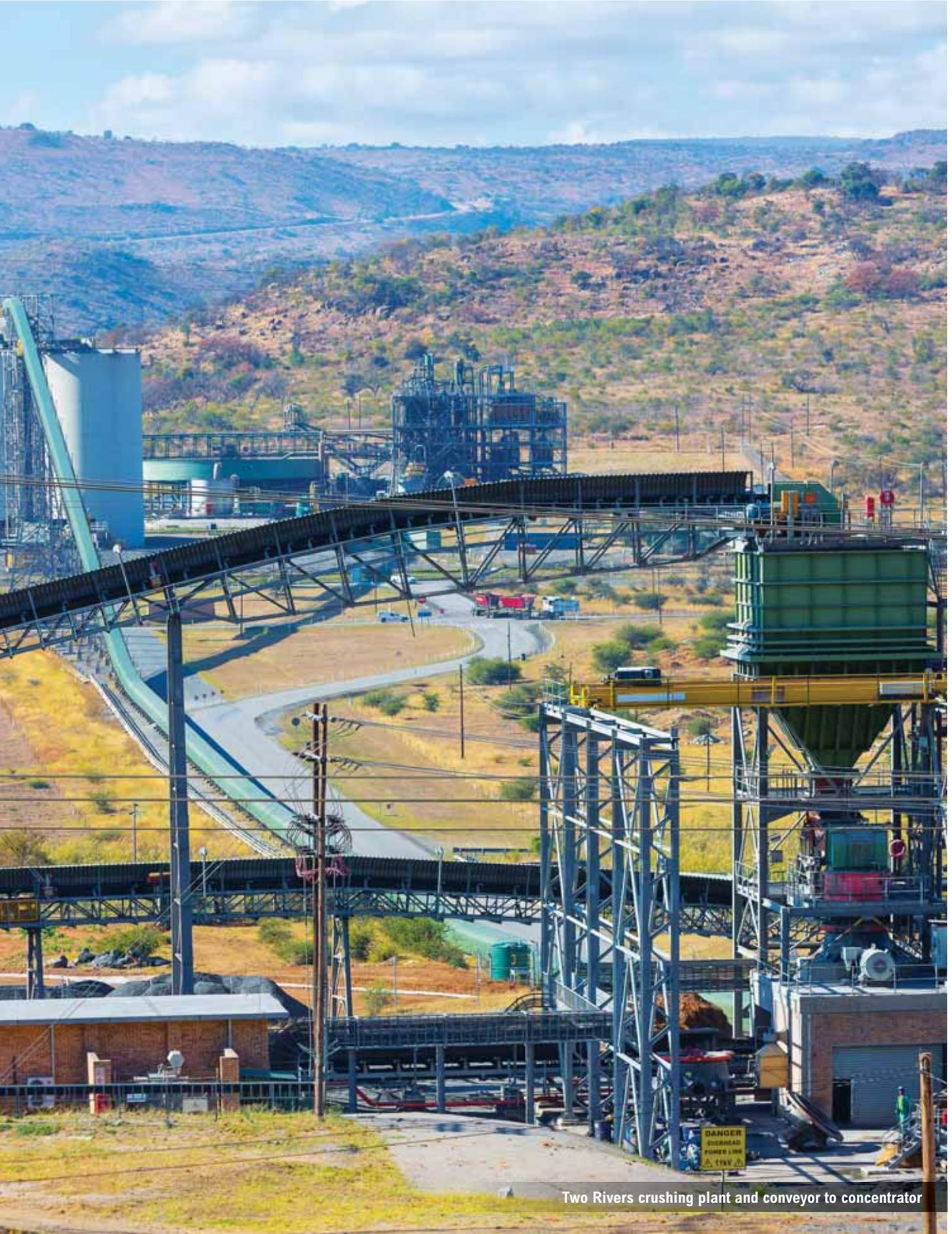
Two Rivers crushing plant and conveyor to concentrator
